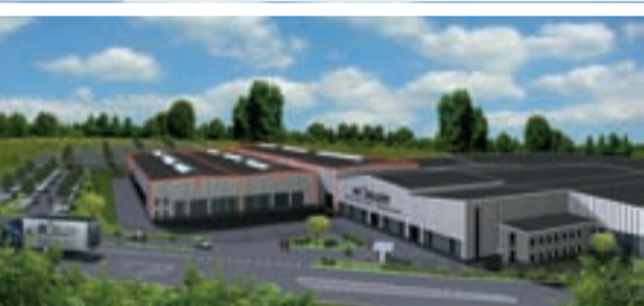
New production areas for the production of shot blast systems at the Untermerzbach site. Completion: August 2007
