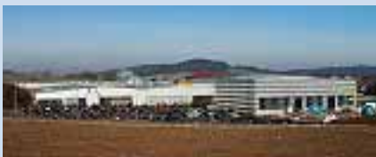
Expanding shot blasting production at Rösler Untermerzbach, Germany
